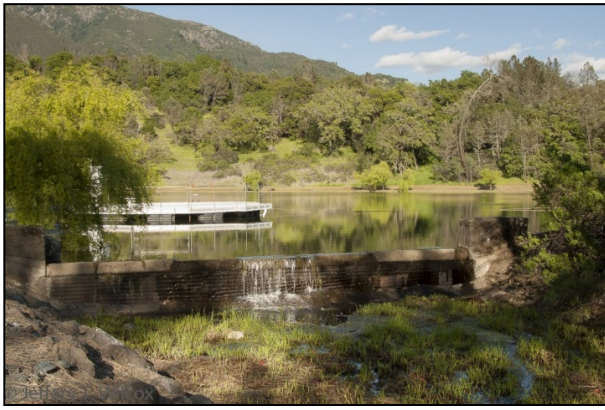
FIGURE 1. Stewart Pond, a reservoir created by impounding three intermittent streams, at the foot (western slope) of Mount Saint Helena in Sonoma County, California. The dam measures approximately 1 m tall and 10 m wide. (Photographed by Jeffery T. Wilcox).
