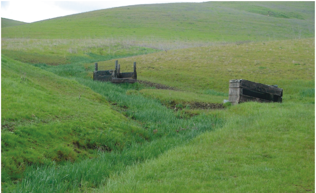
Figure 1. Two typical pre-existing spring boxes placed within a spring in Contra Costa County, California, USA. Each spring box supports California red-legged frog ( Rana draytonii ) adults, and also supports breeding activities and larvae. Pipes from spring boxes allow water to flow down-hill to a concrete trough used to water cattle.
